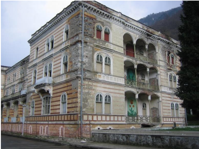
Figure 11: Devasted hotel in the old spa ensemble of Băile Herculane. Photo: JORDAN 2011.
